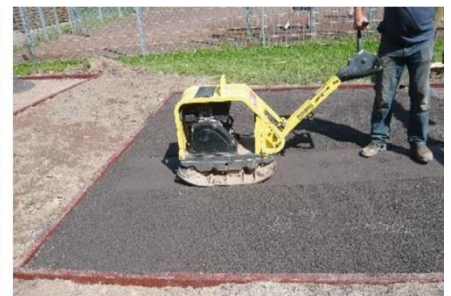
Drainbeton/Splitt standfest verdichten+
